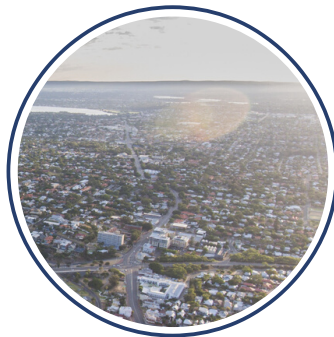
Development and adoption of the Public Realm and Urban Streetscape Style Guide to form consistency and protect the current canopy by diversifying streetscapes.
