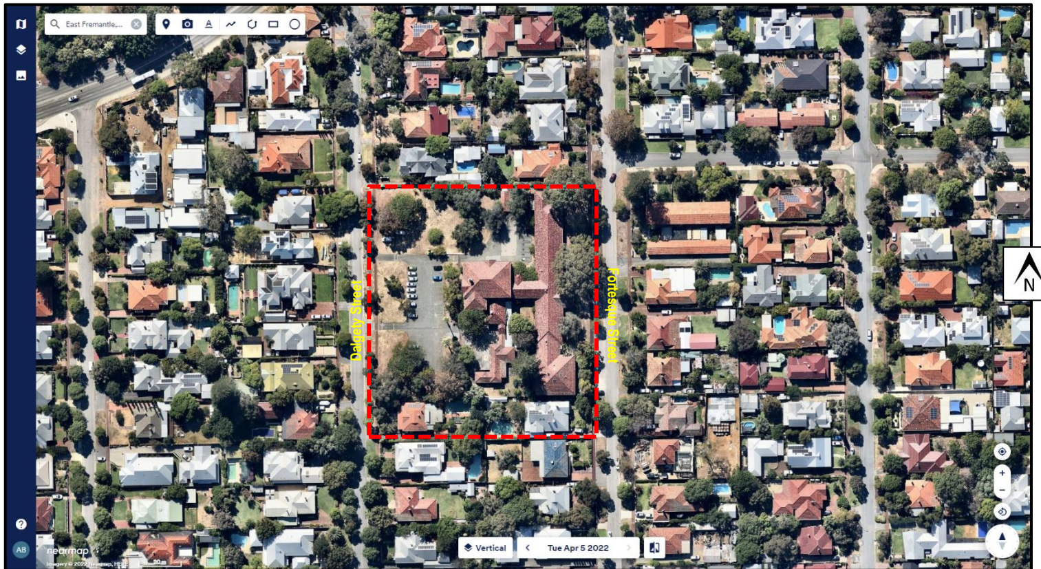
Figure 1. Satellite image showing area of assessment within Woodside Health Care Precinct Upgrade, in East Fremantle, Western Australia. Image Source – www.NearMap.com , Image date 5 th of April 2022
