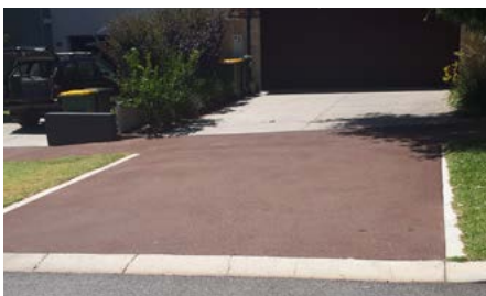
Image 1. Image shows red asphalt footpath and crossover.
