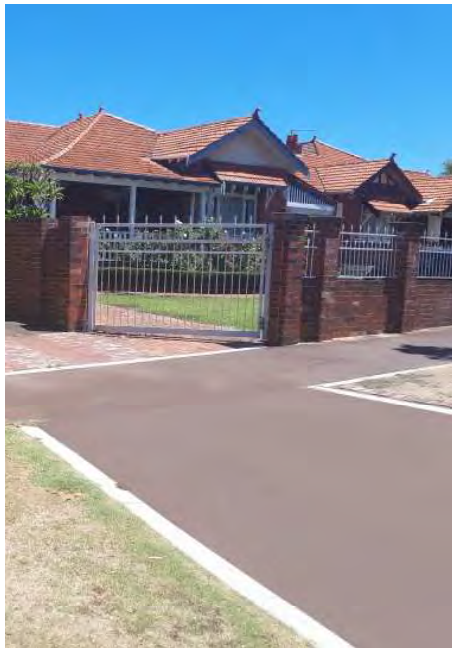
Image 9. Image shows red asphalt footpath priority over residential crossover. Source: UDLA.
