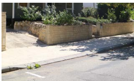
Image 1. Image shows limecrete footpath priority over driveway and crossover. Source: UDLA.
