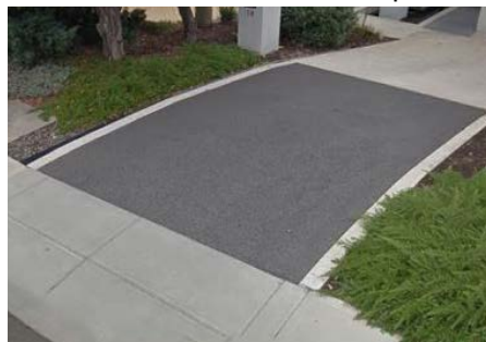
Image 1. Image shows grey concrete footpath priority over driveway and crossover.
